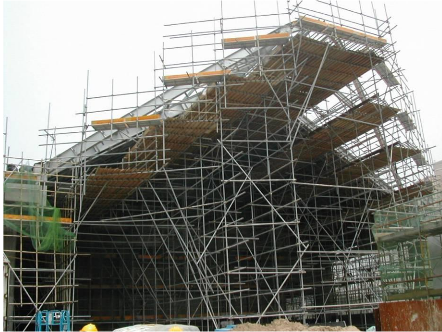
Figure 5.25(d). Ceiling work platforms.
