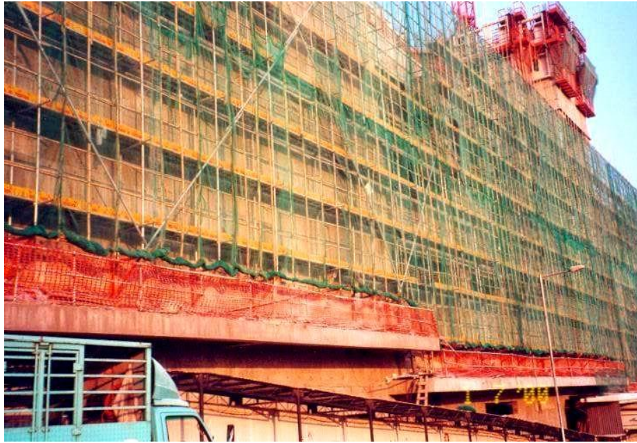
Figure 6.6(b). Work platform of an MBMSS.
