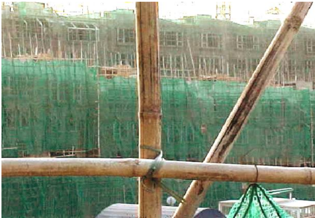
Figure 5.18. Mouldy bamboo in humid conditions.
