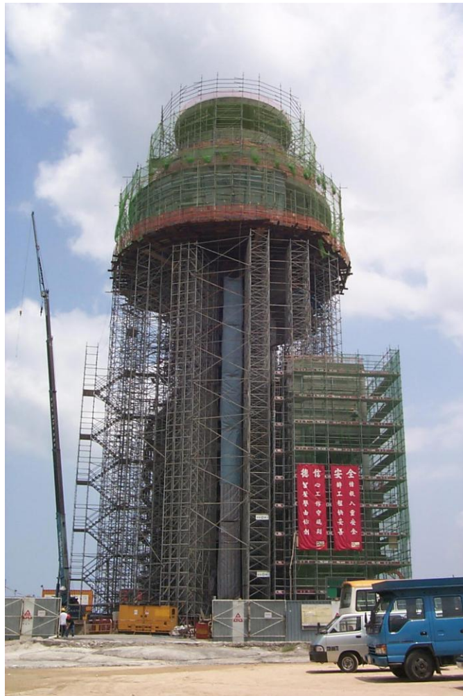
Figure 2.5 Metal scaffold for air traffic control tower.
