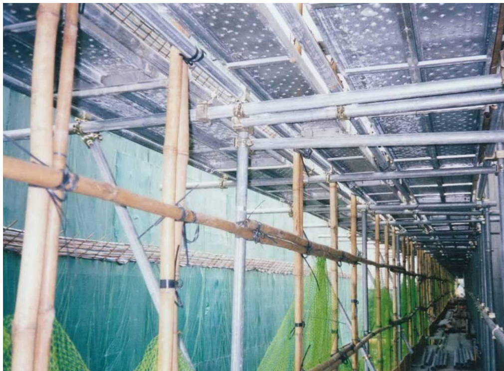
Figure 5.24(b). Cantilever scaffolding.
