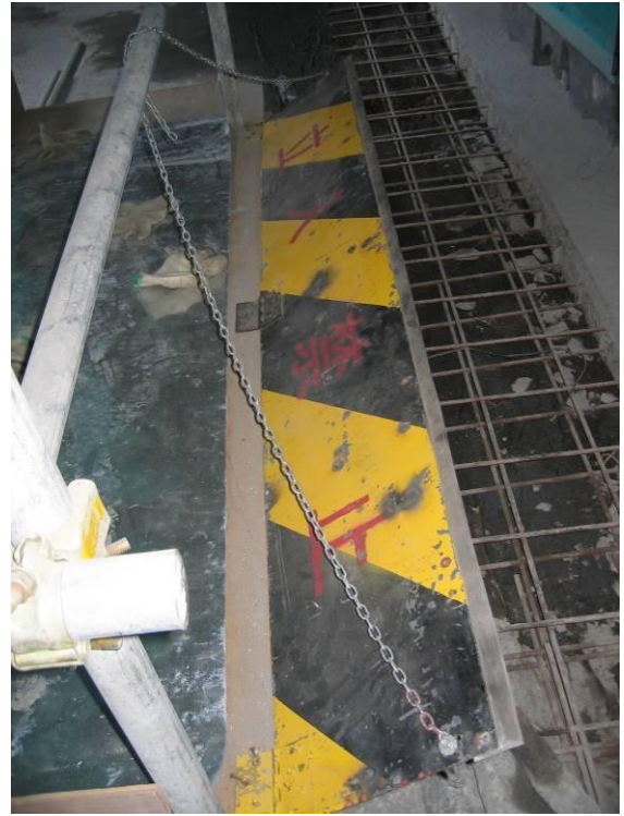
Figure 6.11(g). Movable protective plate.
