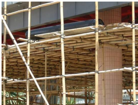
(c) Ceiling platform
