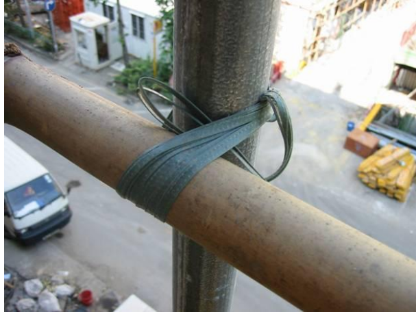
Figure 2.3 Twisting of a nylon tie to secure bamboo and metal tube.
