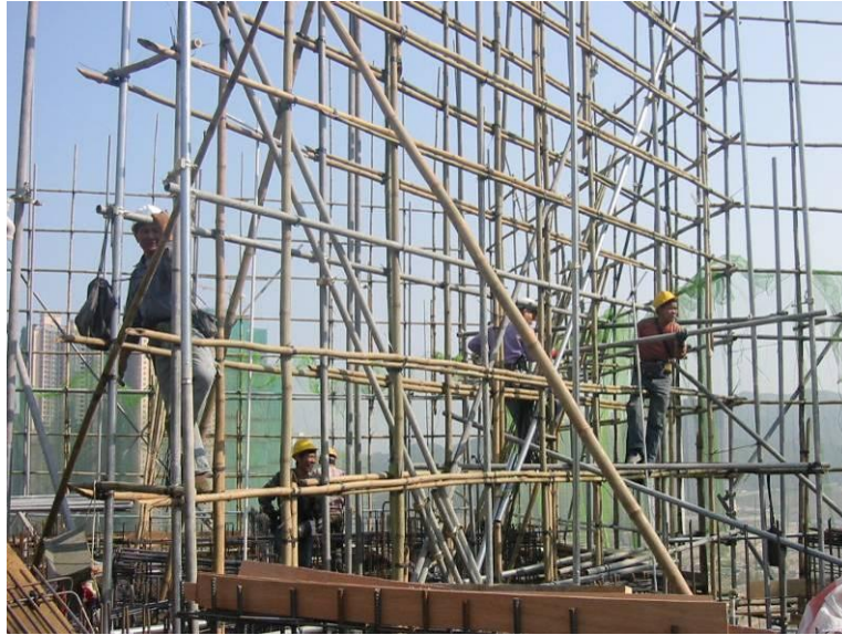
Figure 6.1. Erection of an MBMSS – external façade.
