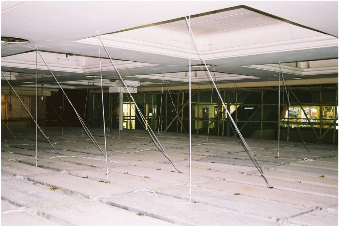
Figure 5.26(b). Surface of the ceiling work platform.
