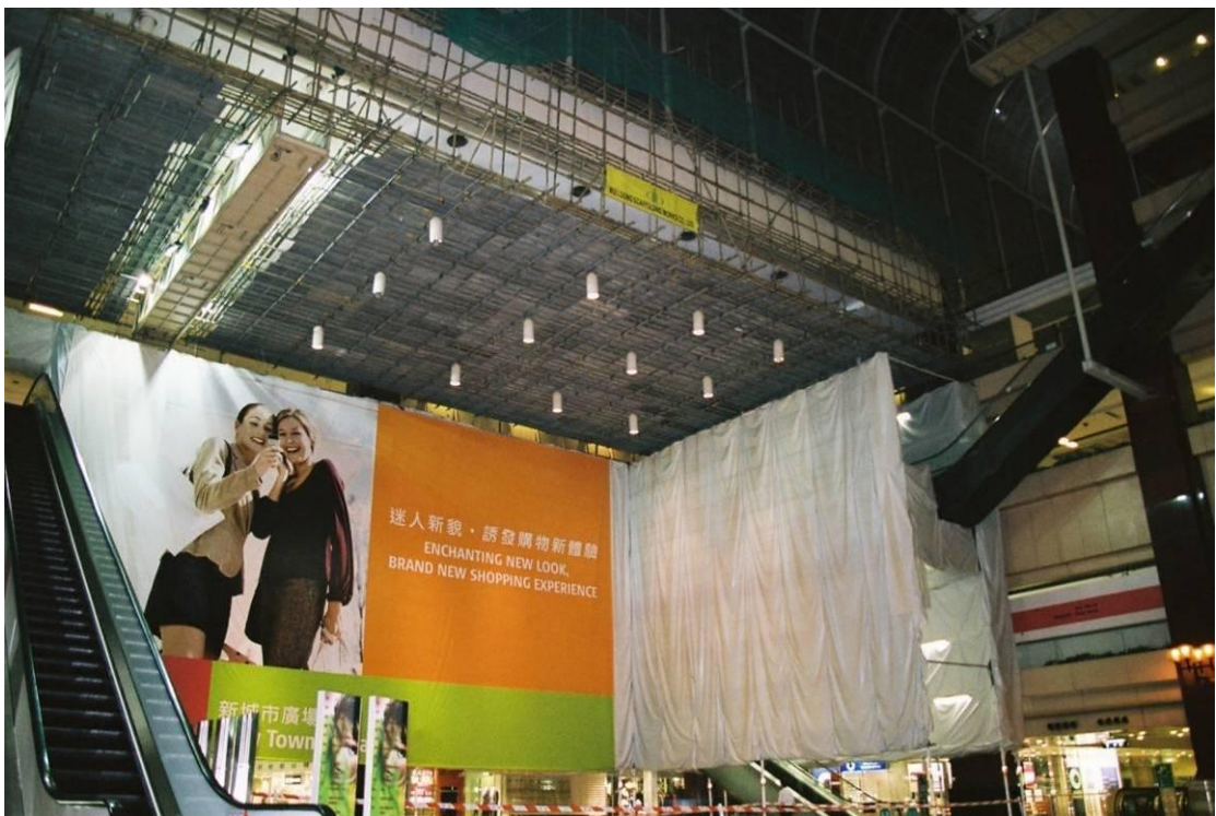
Figure 5.26(a). The suspended ceiling work platform.
