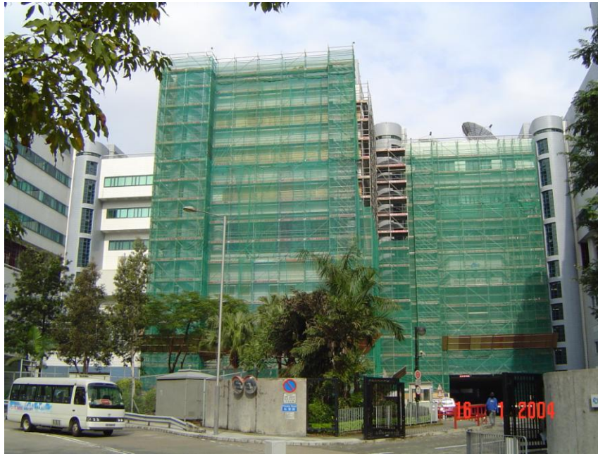
Figure 2.6 Metal scaffold for school rehabilitation project.
