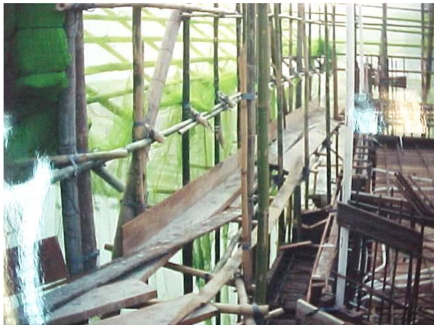
Figure 6.6(c). Work platform/wooden planks of a bamboo scaffold.
