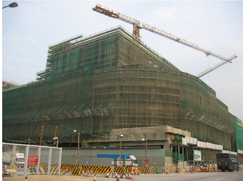
Figure 2.4 Metal scaffold for freight terminal.
