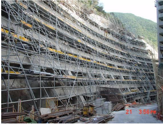
(a) Metal slope scaffold
