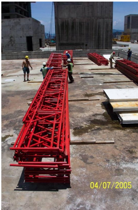
Figure 6.11(a). Frame assembly.
