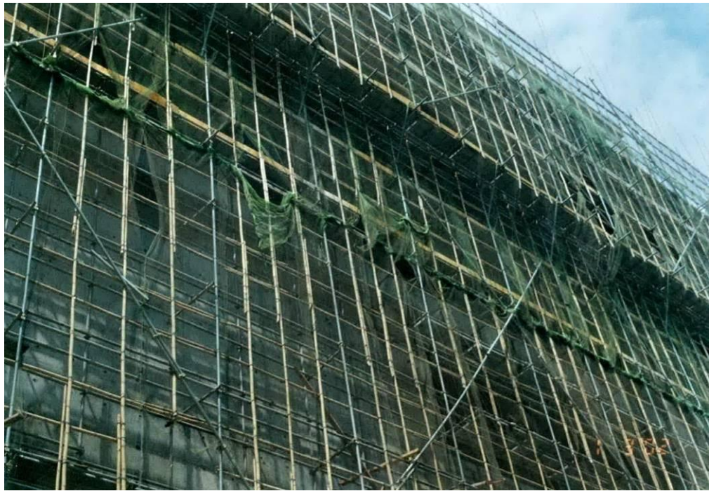
Figure 5.24(a). Cantilever scaffolding.
