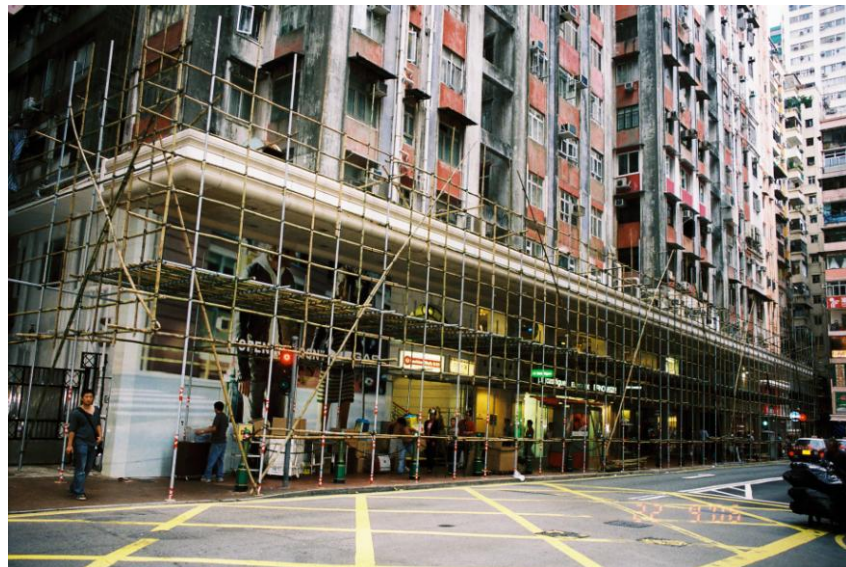
Figure 7.1 A mixed metal and bamboo scaffold
