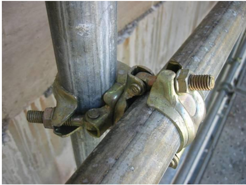
Figure 3.6 Metal coupler connecting two metal tubes.
