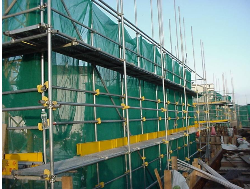
Figure 6.6(d). Wide span of members of a metal scaffold.
