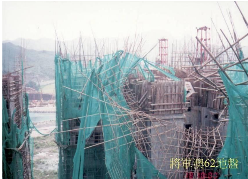
Figure 6.4(a). Bamboo Scaffolding at TKO 62 – 1999.
