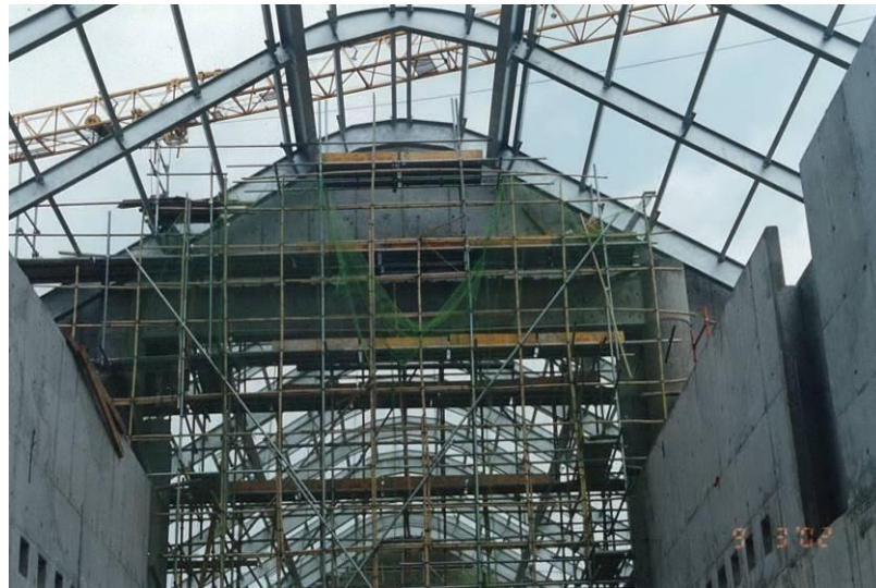
Figure 6.2. Erected MBMSS in a light well.
