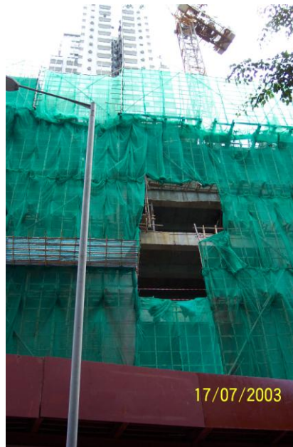
Figure 4.1 Opening in a bamboo scaffold.
