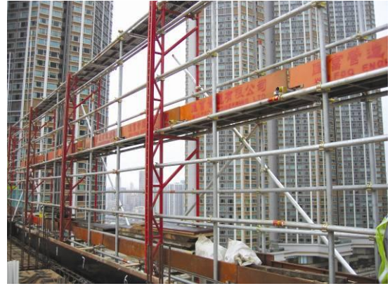
(b) Climbing scaffold
