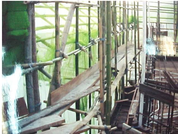
Figure 4.3 Traditional work platform for bamboo scaffolding
