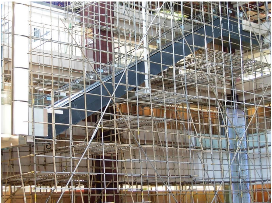
Figure 5.28. Work platforms for the base of an elevator.
