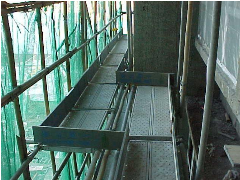
Figure 5.16. Modified inner scaffolding.
