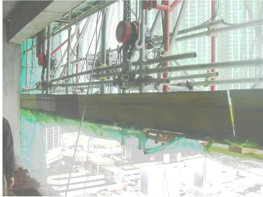
Figure 6.11(e). Side view of the bottom part of the climbing scaffold.
