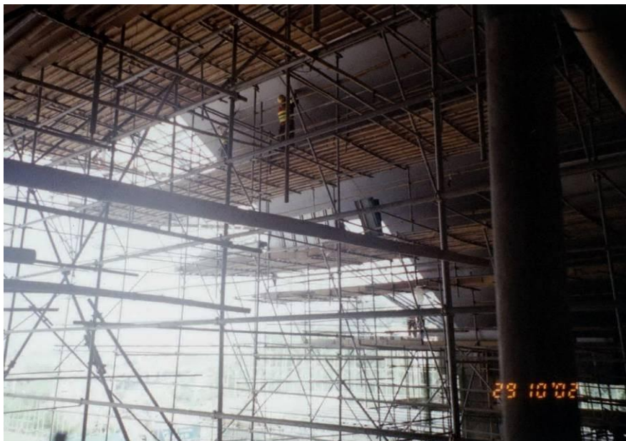
Figure 5.25(c). Ceiling work platforms.
