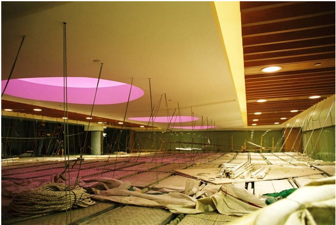
Figure 5.26(c). Surface of the ceiling work platform.
