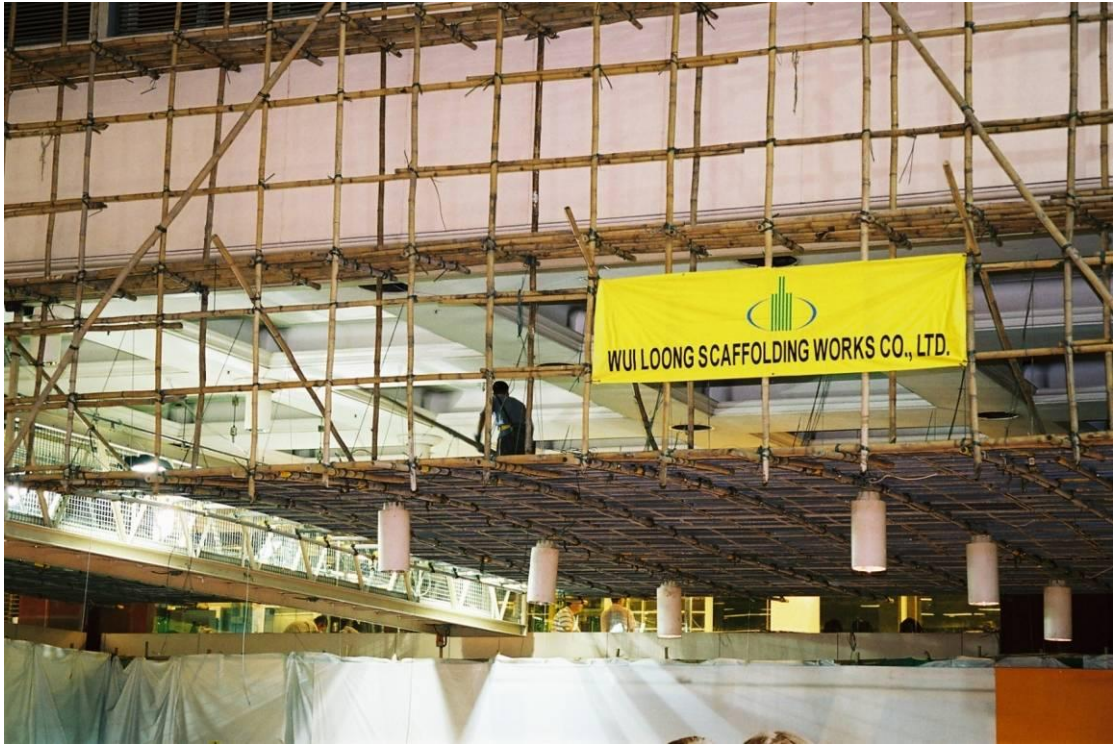
Figure 5.26(d). Surface of the ceiling work platform.
