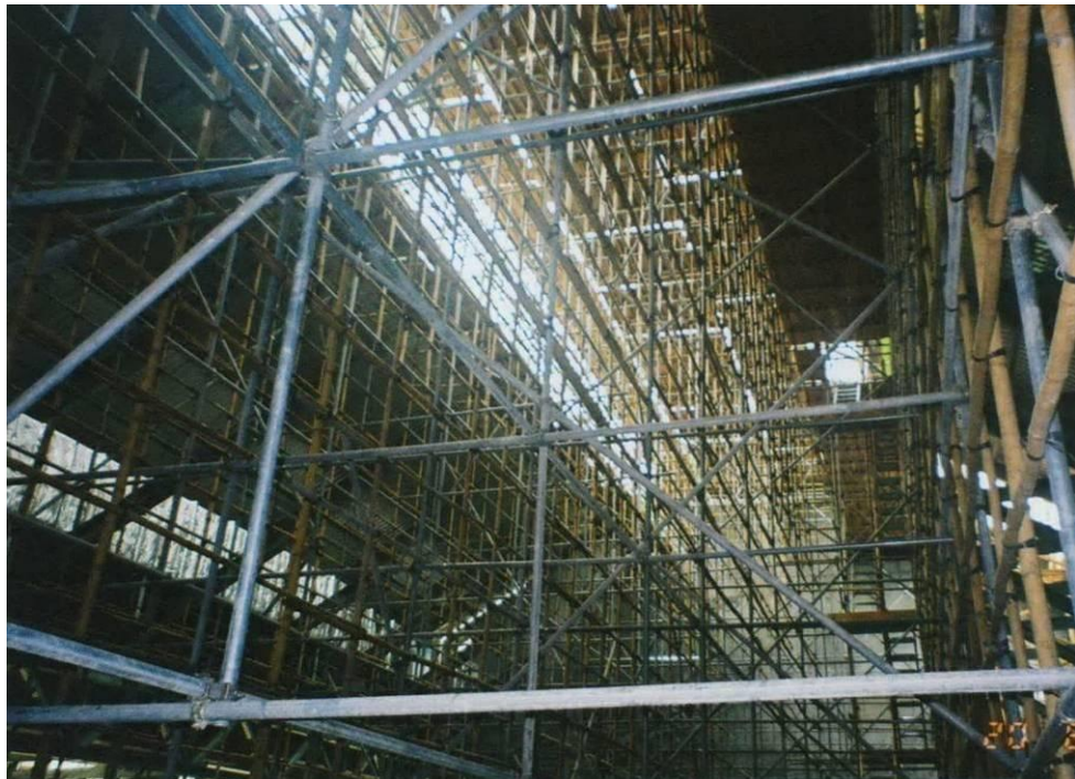
Figure 5.25(a). Ceiling work platforms.
