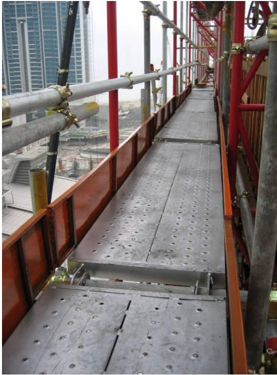
Figure 6.11(f). The work platform and toe-board.
