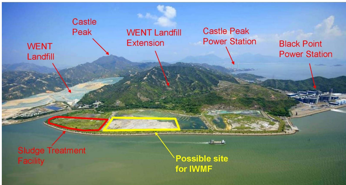
Figure 3.5: Proposed location of IWMF in Tsang Tsui Ash Lagoons sites in Tuen Mun
