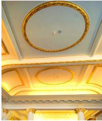
Photo 5-18 Ceiling smoke detector
