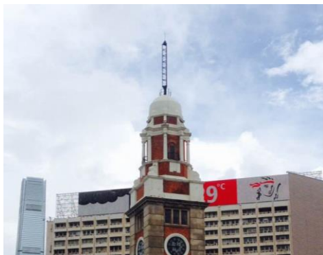
Photo 5-22 Lightning rod of the Clock Tower
